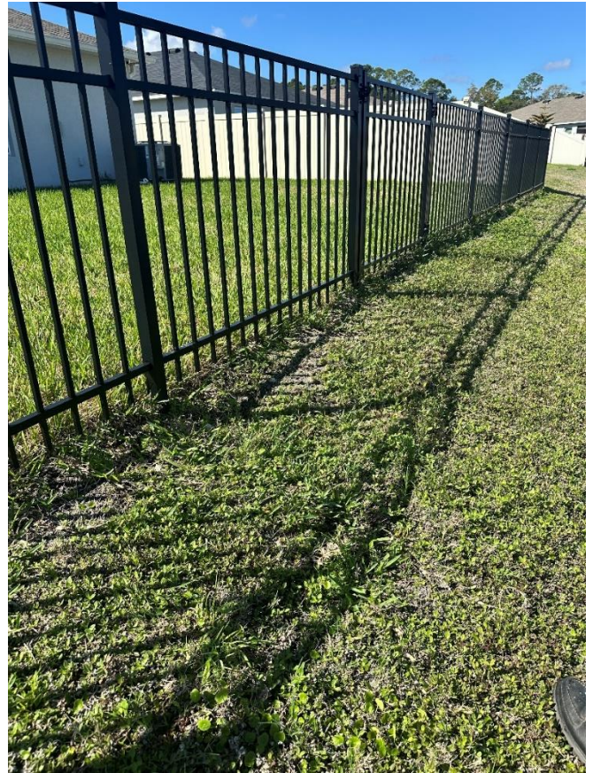
Photo 10. 1290 Moscato Lane rear.
