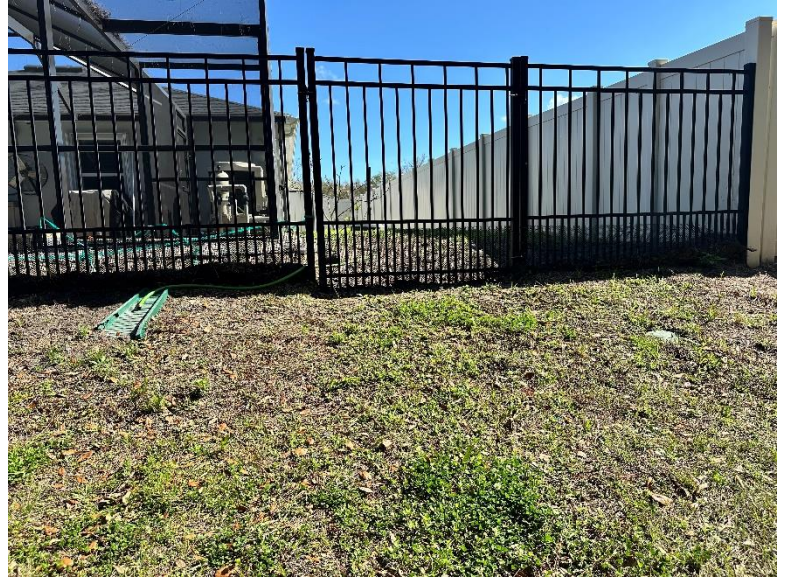
Photo 2, 1399 Moscato Drive east rear corner.
