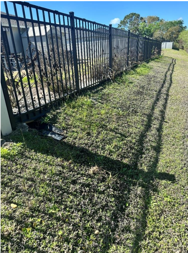
Photo 17, 7694 Fortana Way rear showing piped roof drains.
