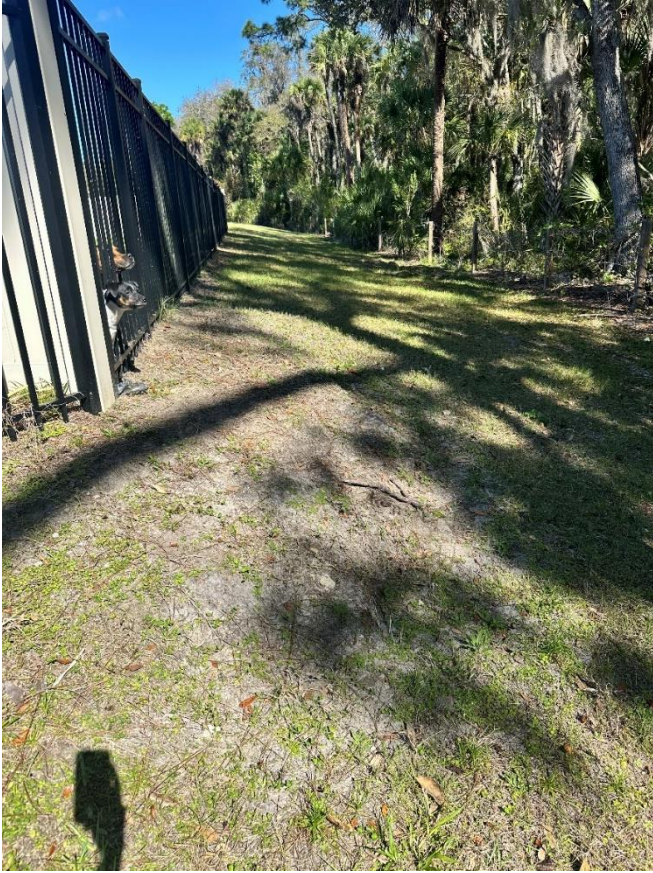
Photo 7. Corner between 7701 and 7711 Prosecco Lane.
