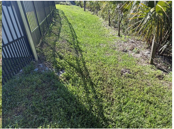
Photo 8. Rear of 1671/1661 Pecorino Court.
