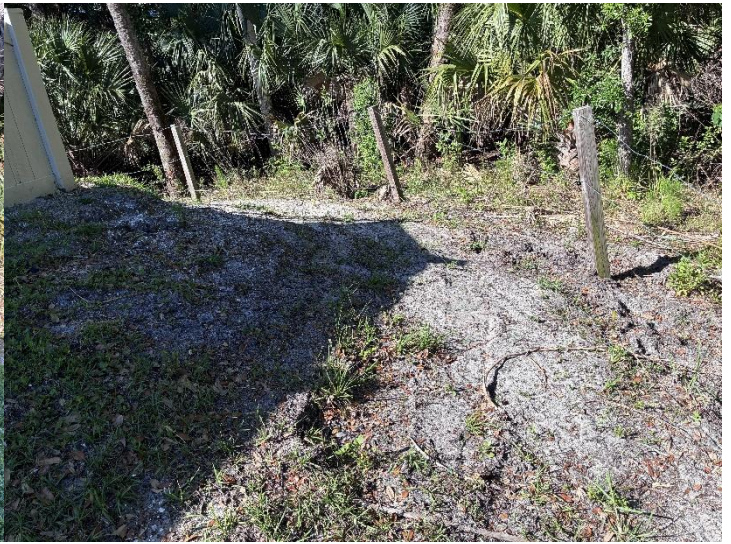
Photo 2. Corner of 1711 Pecorino Court.
