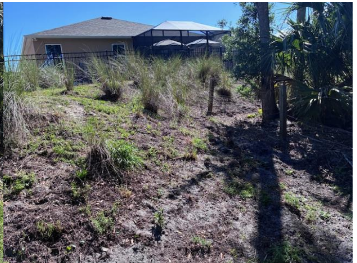
Photo 12. Rear of 1631 Pecorino Court.
