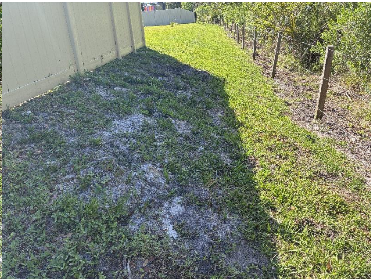
Photo 6. Rear of 1701 Pecorino Court.
