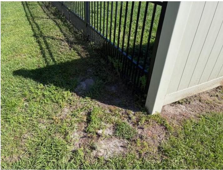
Photo 15. Rear of 1621 Pecorino Court.
