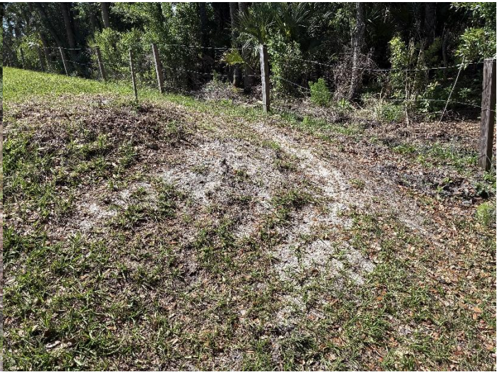
Photo 58. Corner of 1461 Pecorino Court.
