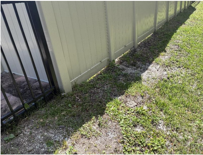
Photo 55. Rear of 1501/1491 Pecorino Court.
