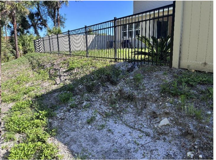
Photo 4. Rear of 1711/1701 Pecorino Court.
