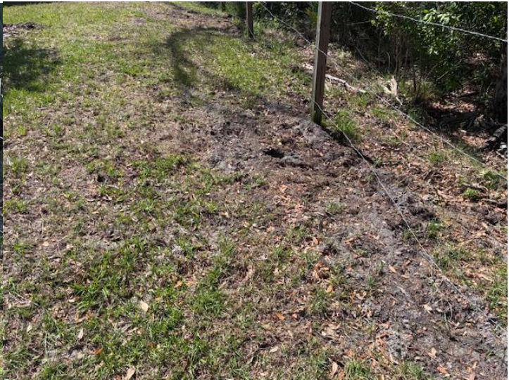
Photo 60. Rear of 1451 Pecorino Court.
