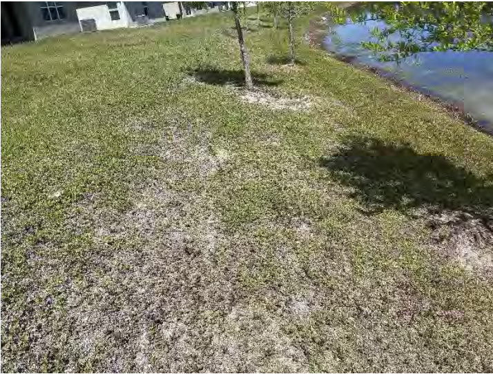
Photo 77. Rear of 1652 Pecorino Court.
