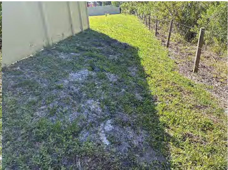
Photo 6. Rear of 1701 Pecorino Court.
