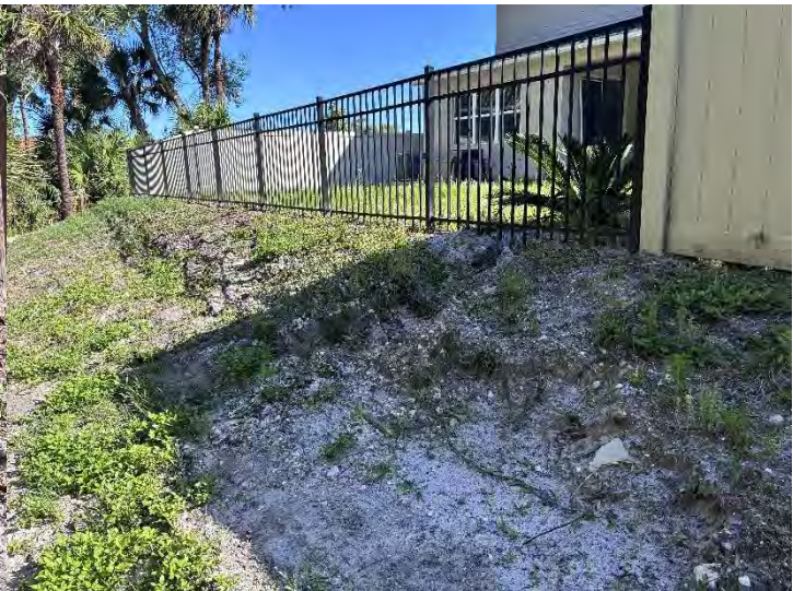
Photo 4. Rear of 1711/1701 Pecorino Court.
