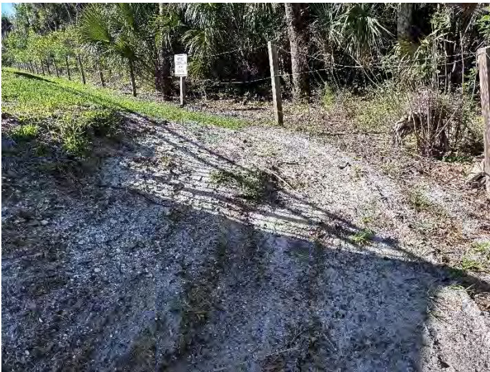
Photo 3. Corner of 1711 Pecorino Court.
