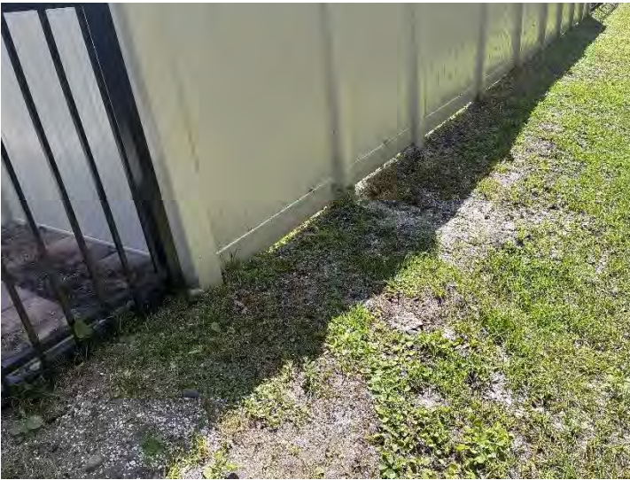
Photo 55. Rear of 1501/1491 Pecorino Court.
