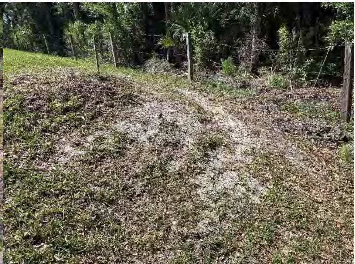
Photo 58. Corner of 1461 Pecorino Court.
